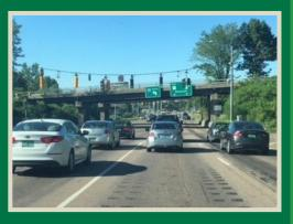
The current interchange at Exit 16 is a grade separated tight diamond interchange with I-89 crossing over US Routes 2/7 via two bridges. The existing interchange yields frequent traffic congestion, lengthy delays, and significant queuing during peak hours. These existing conditions are a safety concern with a high number of incidents, collisions, and a lack of accommodations for nonmotorized travel.
